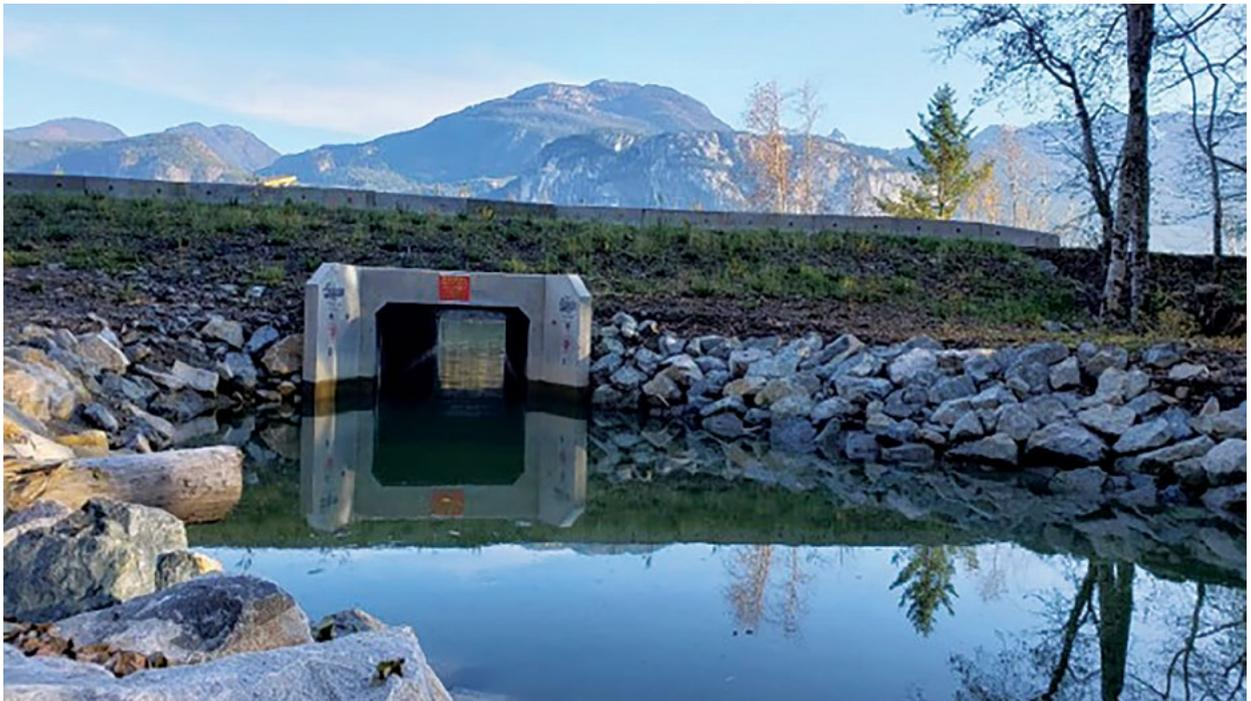
A box culvert installed in the dike to increase connectivity between the Squamish River and the estuary. (Credit: Edith Tobe)
