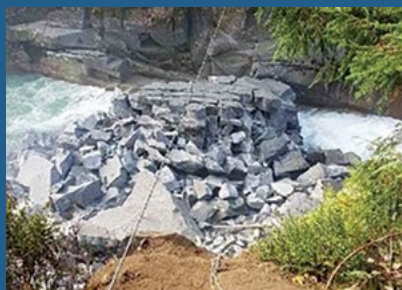
The boulder after it had been blasted apart.
