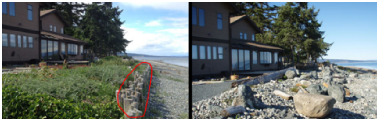
A Green Shores project on an eroding shoreline in Qualicum Bay, Vancouver Island. Left – before restoration. The red line encircles a failing wooden bulkhead where erosion was beginning to undermine the structure. Plants were non-native species. Right – after restoration. The wooden bulkhead was removed, and the shore was regraded to a more natural slope. Large boulders were placed at ~1 m depth and infilled with smaller rock, sand and gravel, to provide a growing medium for native plants. Logs were buried along the upper portion of the shore to mimic the natural shoreline and provide shelter for plants to grow (Photo credit: Green Shores).
